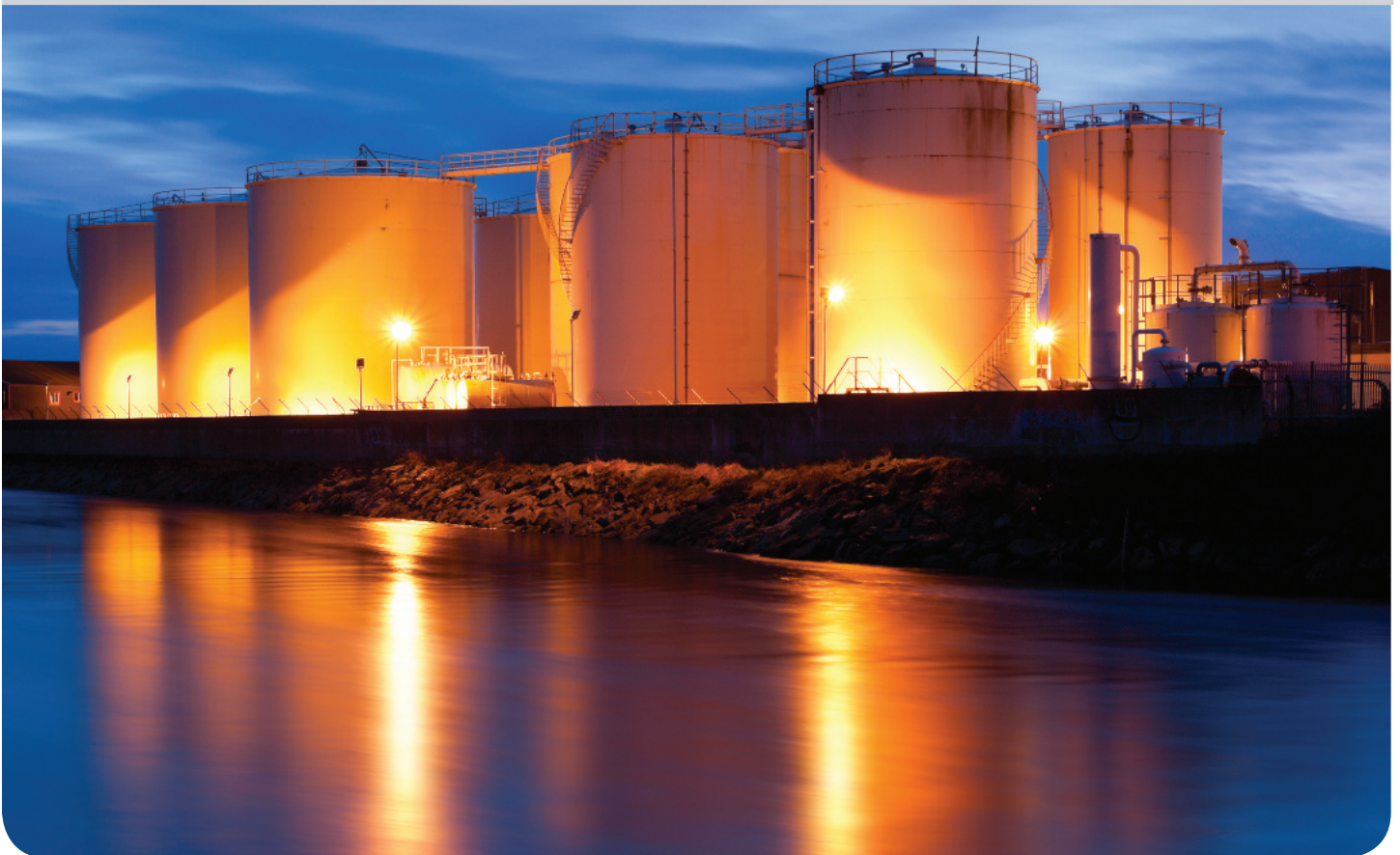
Chemical tanks in remote locations can pose extensive monitoring challenges.
